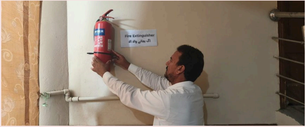
An inspection officer of the Commission checking a fire extinguisher
